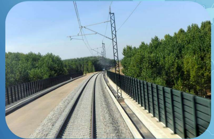
High Speed Line network in Spain opened to public in 2022
