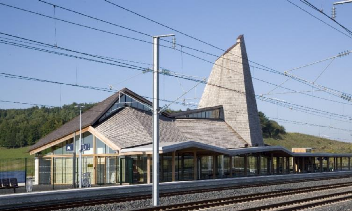
Meuse High speed station –Wood building
